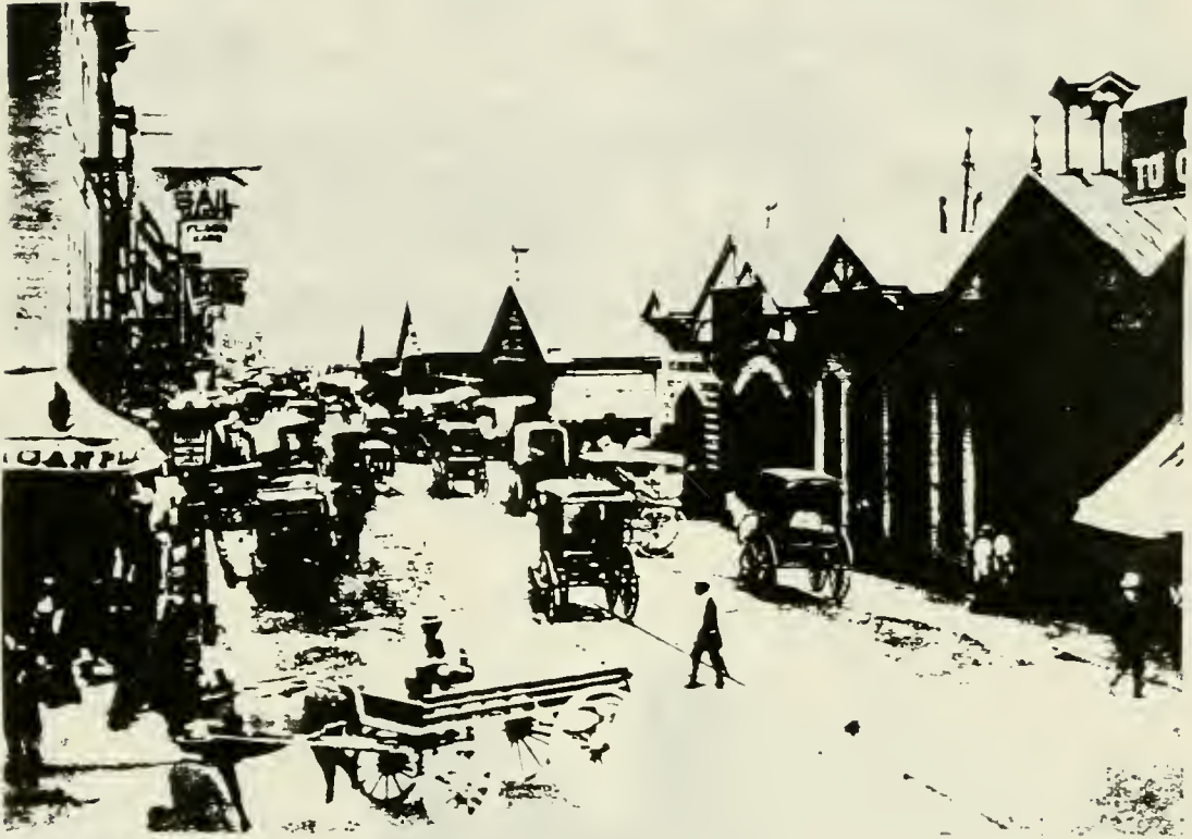
FIGURE 2.1 Delaware Avenue Looking North from Market Street, circa 1890. From Looney, Old Philadelphia in Early Photographs .
